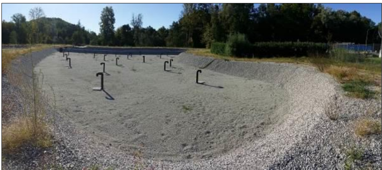
Figures 2 – The submerged flow basins at the current date
